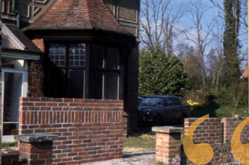
Clockwise from left to right: THE LANDMARK CRANES viewed from the Corner of Adams Road in 1978 THE ENTRANCE RAMP finally takes shape (7-1980) THE HALL begins to take shape (3-1978) TEST PANELS OF BRICKS built around the patio at Thorneycreek to appraise how the all-brick building might finally appear – (2-1976)
